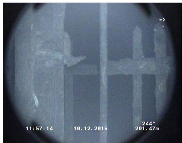
Fig. 3 Gate at the 200 m Level in a video record of the flooded Wolf Mine shaft. The still image was taken at a camera depth of 201.47 m below shaft collar or 121.5 m b.w.t
